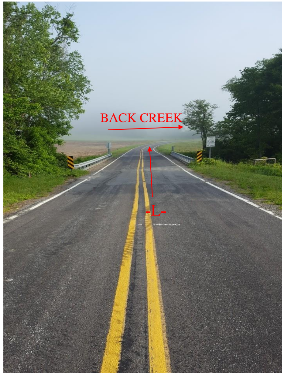
Photograph No. 1: At End Bent 1 looking towards End Bent 2
