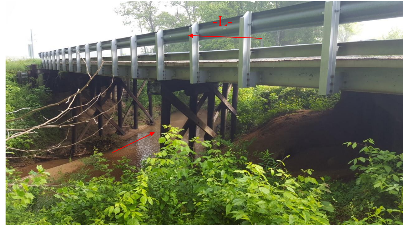
Photograph No. 2: Looking Downstream
